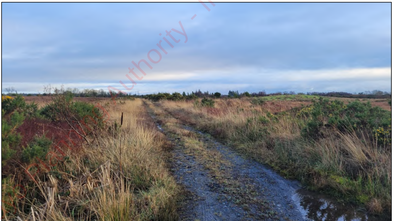
Photo 2: Existing Site Track to be Upgraded
